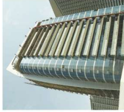
DUBAI-Oasis 1 & 2 Tower Investors - Dubai Sports City
